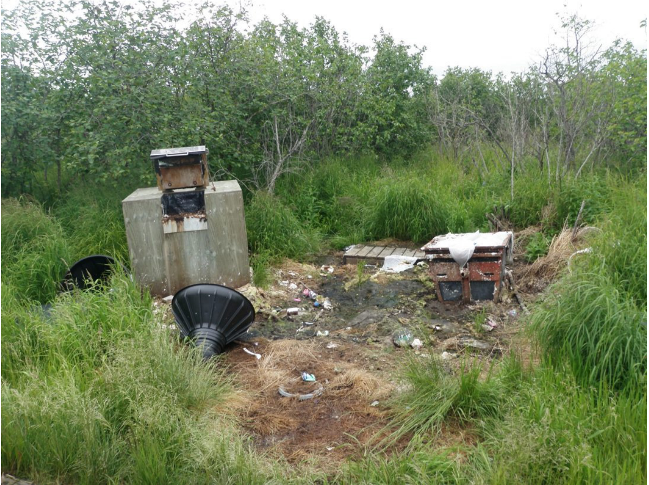
Example of a centralized disposal bunker and dumpster for village in-home 'honey bucket' waste. A honey bucket is a bucket that is used as a toilet in communities that lack a water-borne sewage system. Image courtesy of The Rural Alaska Water and Sanitation Working Group.
