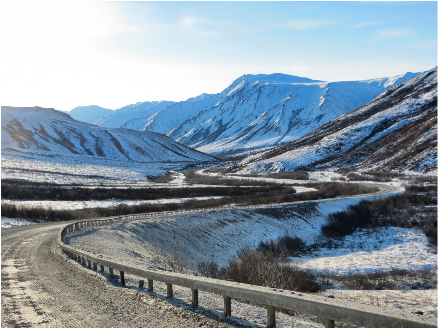
The USARC Goals Report identifies frozen debris lobes (slow-moving landslides) as a potential threat to the infrastructure of the Dalton Highway in the Brooks Range, Alaska. Image courtesy of Scott McMurren.
