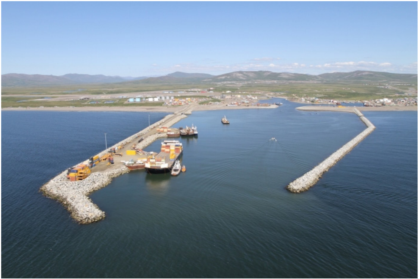
In its 2015-16 Goals Report, the USARC encourages additional civil engineering research toward developing a system of deep." Port of Nome, Alaska is pictured here. Image courtesy of the U.S. Army Corps of Engineers.
